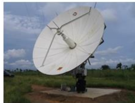
Backhaul site, Lobito
